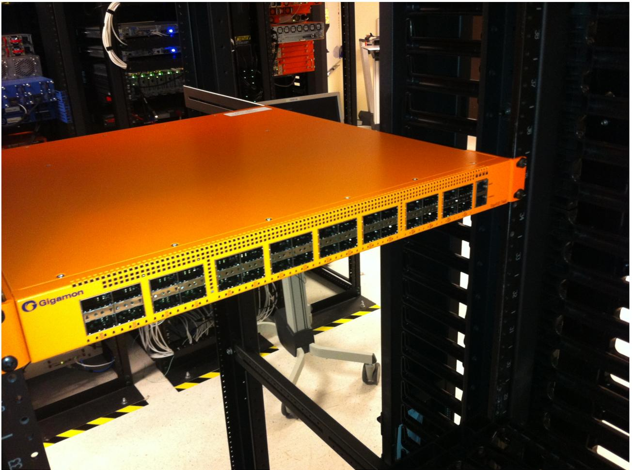
**Figure 12** *Front View of the Mounted Node to the Four-Post Rack*
