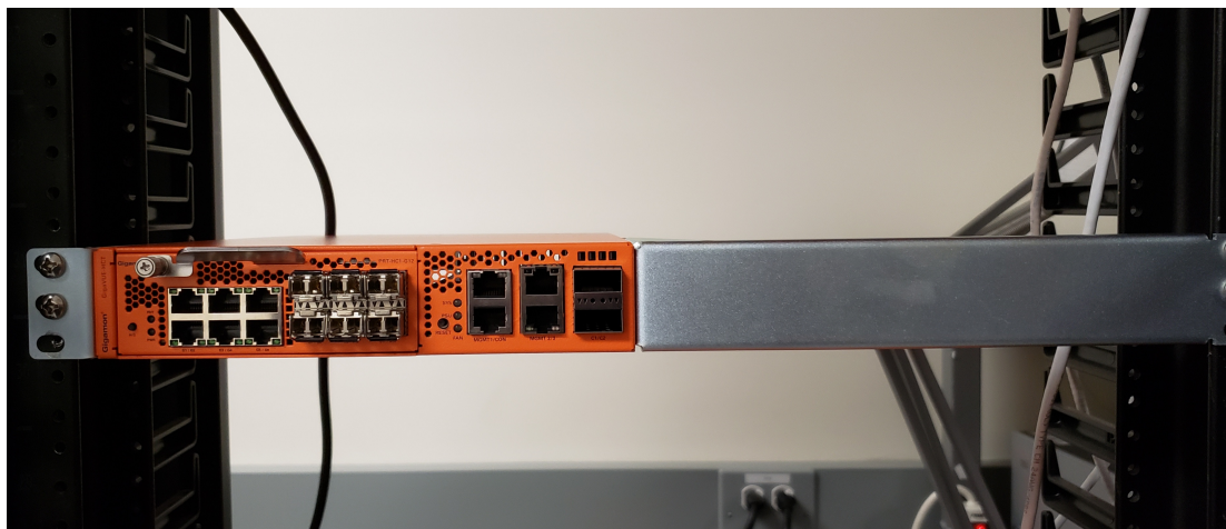
Figure 10 Four-Post Rack Installation (Single Chassis Assembly)
